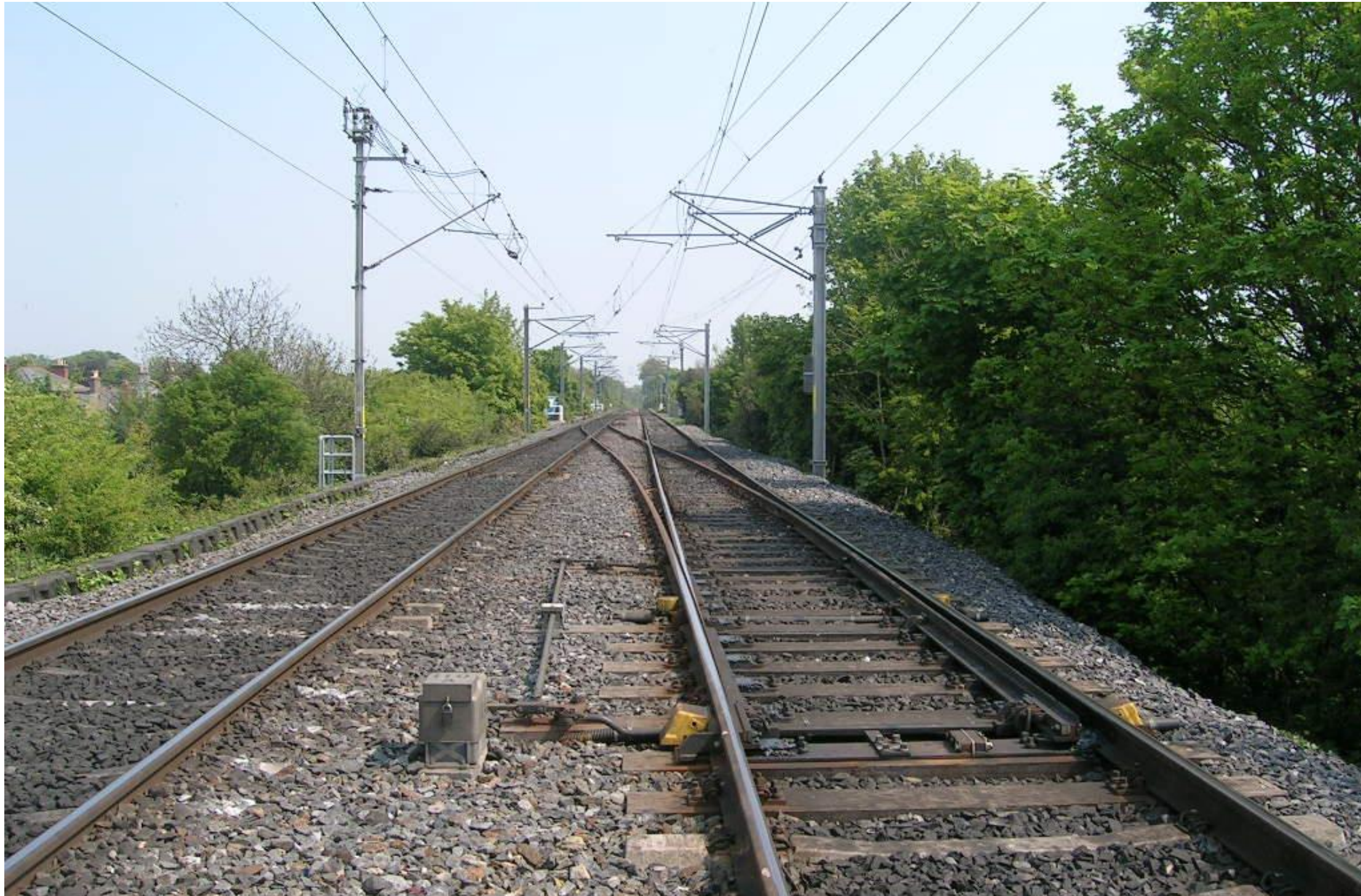
View of typical section of twin track electrified rail line
