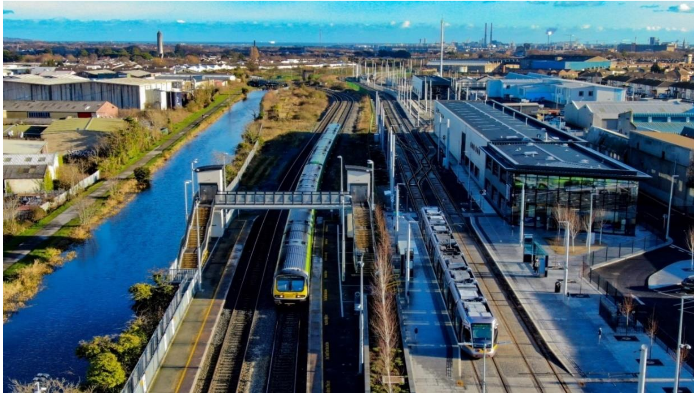
Aerial view Broombridge integrated rail and LUAS stations
