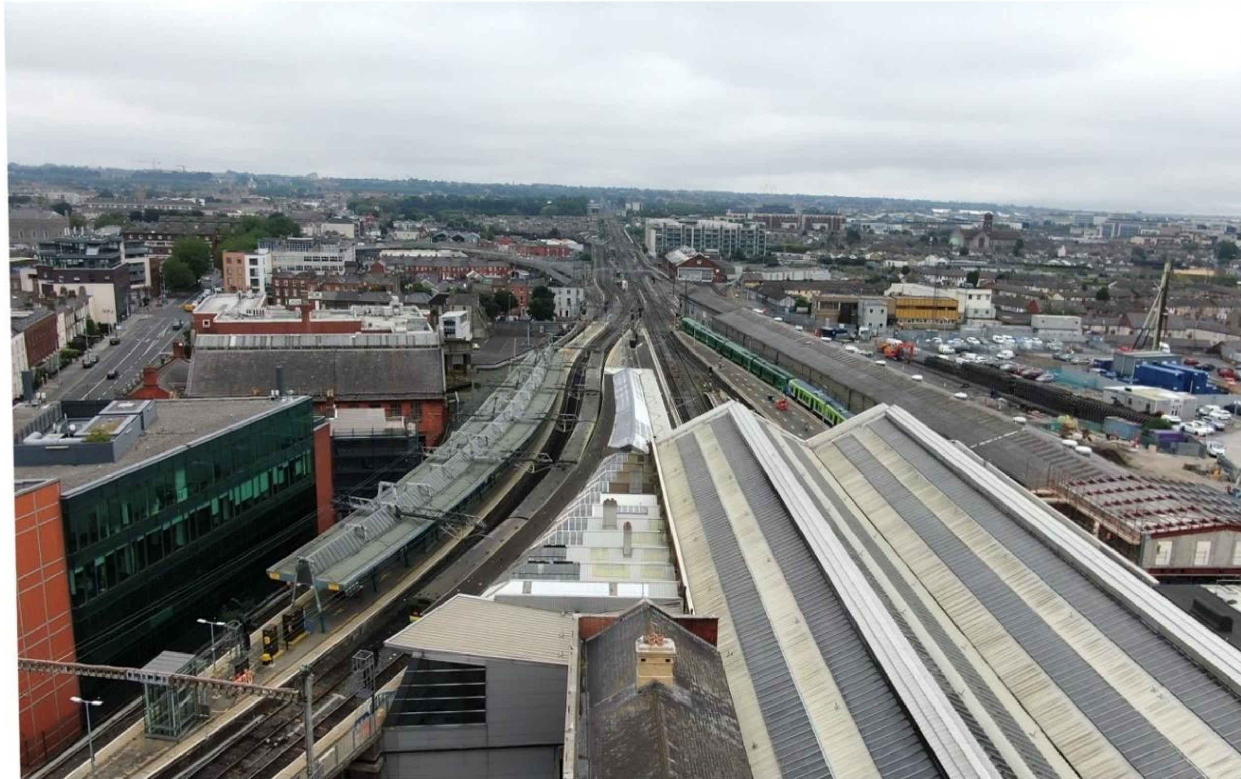
View of tracks on northern approach to Connolly Station showing multiple crossovers which restrict capacity
